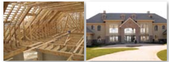
Attic roof structure
