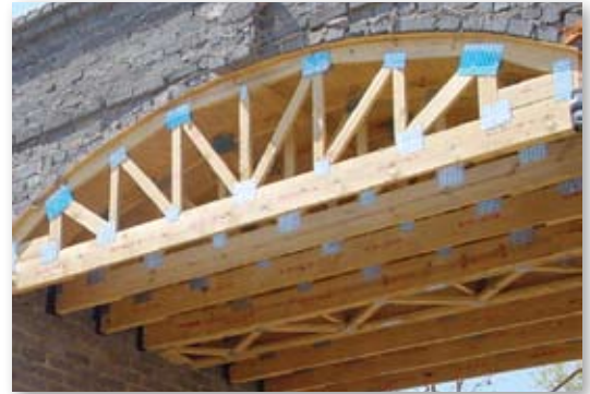
Form-work truss for bridge construction
