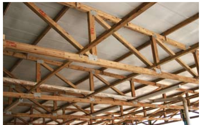
MiTek Industries' nail plate can be seen in the Biligom® in a roof structure
